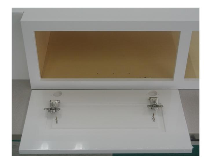
Fine punch holes are given on frame as guidance for hinge mounting. However verify punch hole carefully at 2-9/16" as shown and attach hinges to side of face frame.
