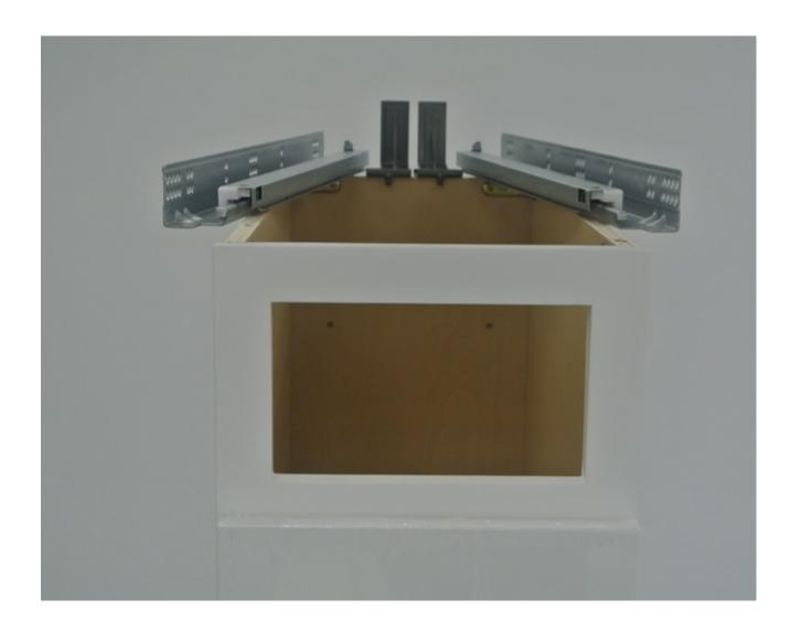
Insert each rear slide support in the two holes and screw to the back panel.
