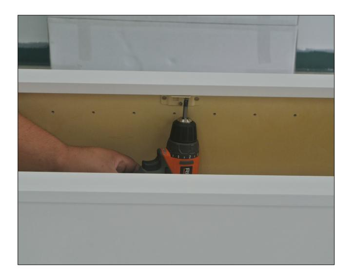
Install Brackets A on face frame and sides.
