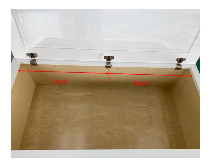
Attach hinges to side of face frame. Ensure screw in the exact center of hinge hole.
